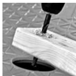
Bohrloch / Hole for drilling
